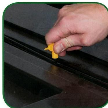
Using the holer puncher fit the connection nozzle into pierced holes
